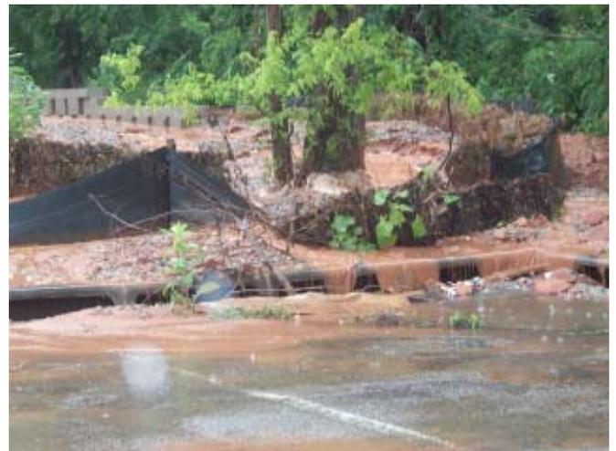
**Pictured is a storm water complaint resulting from a discharge at a construction site.**
