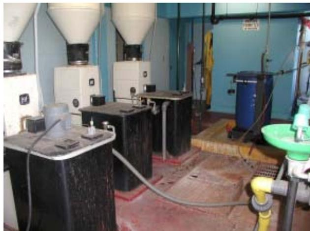
Pictured here are fluoride and polymer feeders evaluated during an inspection.
