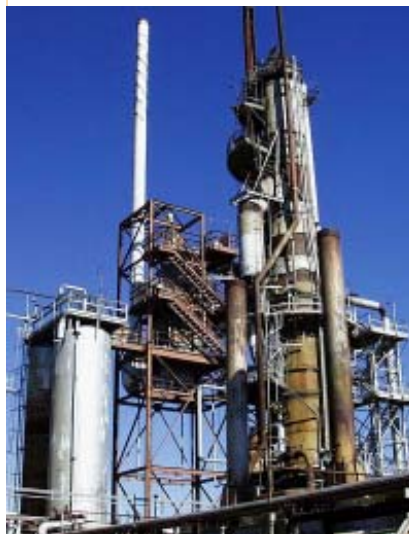
Hudson Refinery structures
