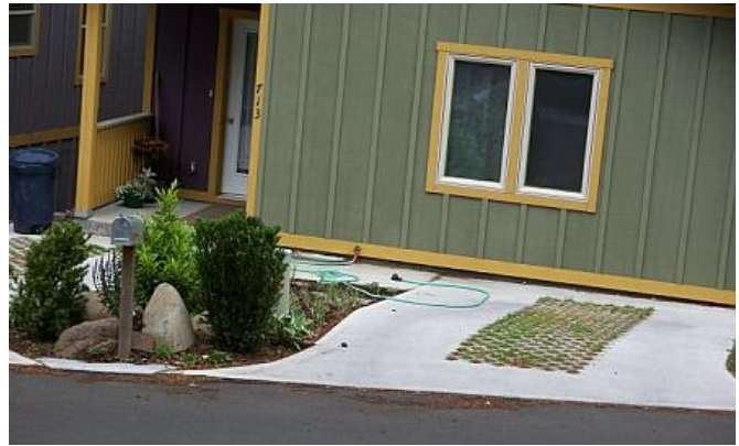
Green driveways and rain gardens are attractive ways of reducing runoff from paved areas.
