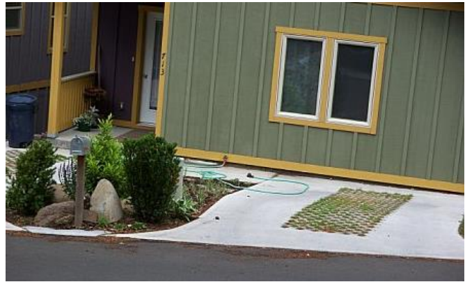
Green driveways and rain gardens are attractive ways of reducing runoff from paved areas.
